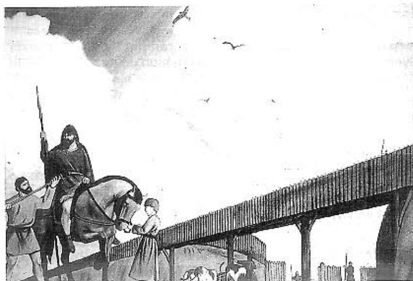
♦ Reconstruction drawing of the entrances from the north by Paul Francis (courtesy of Waterways Visitor Centre, Ringsend)
