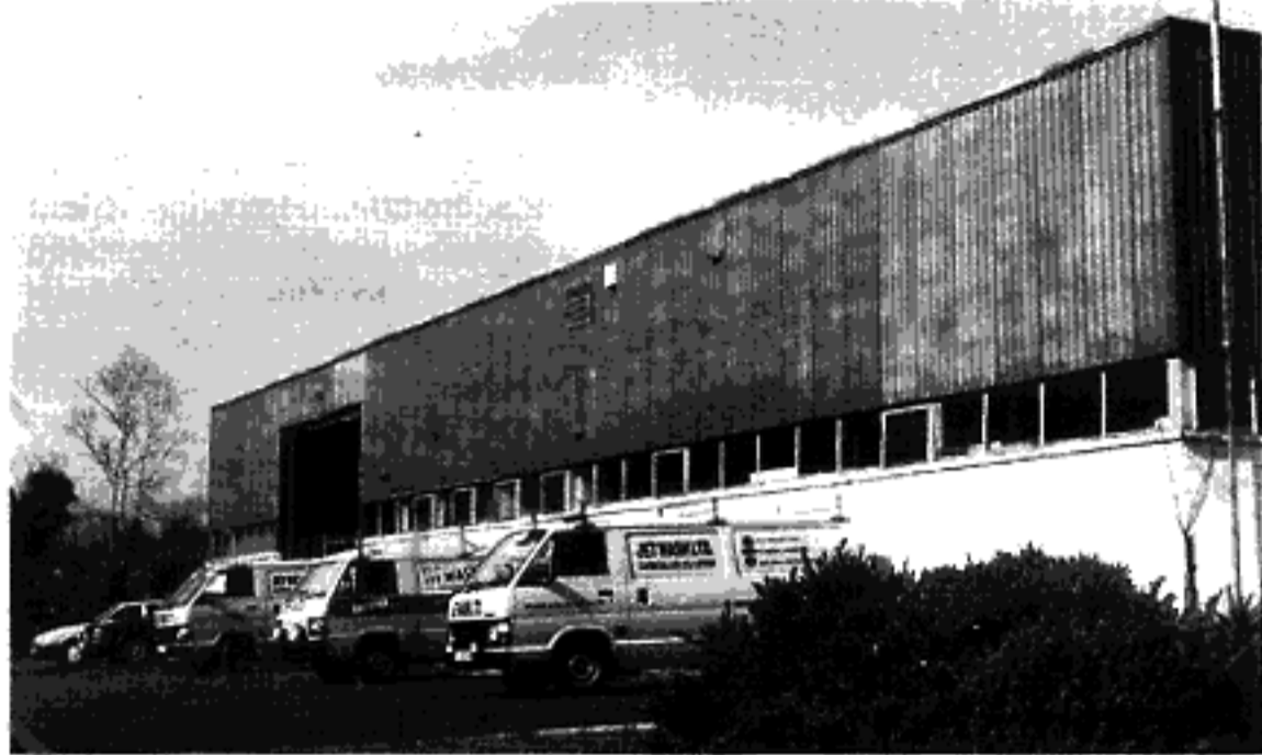
The Jet Wash factory, Carrigallen.
